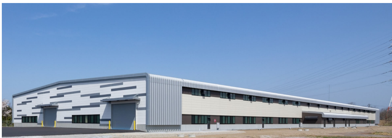
Fukui Yodoko No.2 Plant (No.1 Building)
