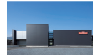
A building with YODO fire-proof panel Grand Wall
