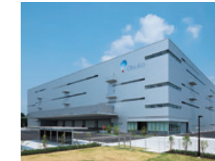
A building with YODO fire-proof panel Grand Wall
