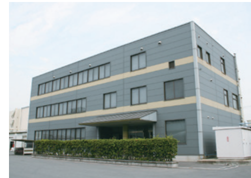
Product Development Center (Osaka Plant)
