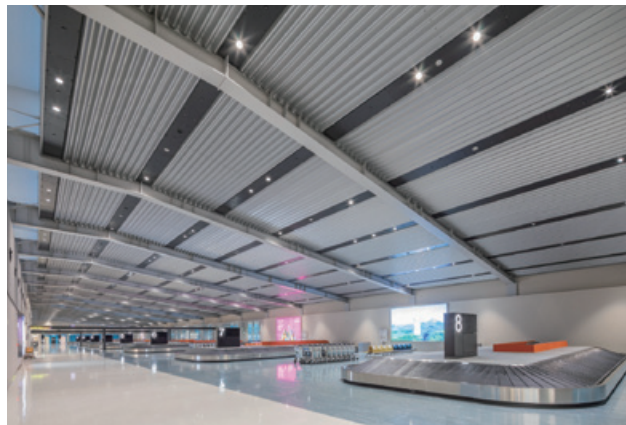
YODO Roof is used in the ceiling of the central terminal at Osaka International Airport
