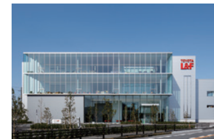
A building with YODO fire-proof panel Grand Wall
