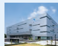
YODO fire-proof panel Grand Wall installation example
