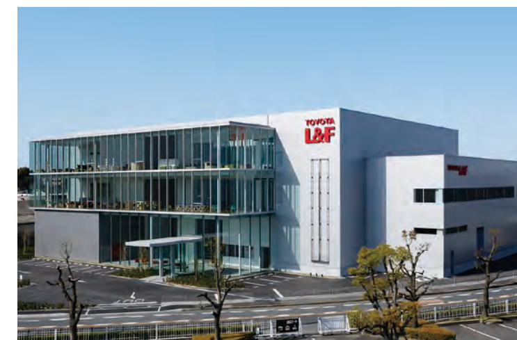
YODO fire-proof panel Grand Wall installation example
