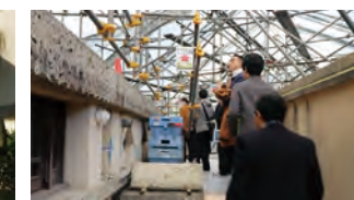
A tour during construction
