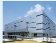
YODO fire-proof panel Grand Wall installation example
